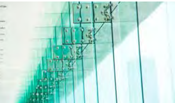
Glass beam lamination without mechanical fixation
